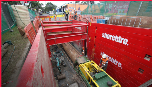
HYDRAULIC BRACING
