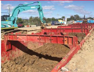
Shore Hire has an Arch Spreader system that integrates with Shore Hire's large range of Steel and Aluminium Trench Boxes, allowing 2500mm of under strut clearance with widths up to 6.5m or more, pending engineering requirements.
