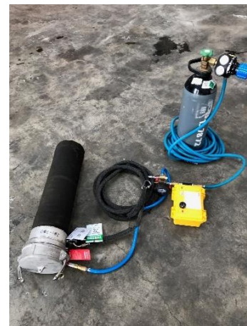
Critical Air Cylinder and Alarm set up
